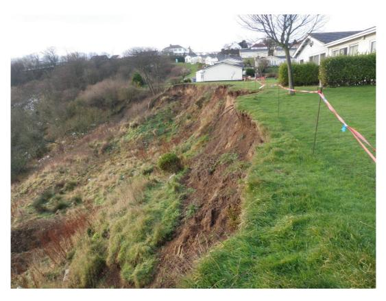
Plate 7 Cliff recession at Knipe Point Headscarp (13<sup>th</sup> December 2010)
