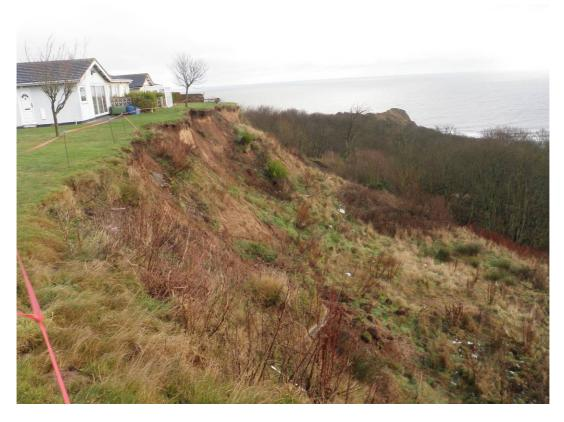
Plate 15 Cliff recession at Knipe Point Headland looking east (13th December 2010)
